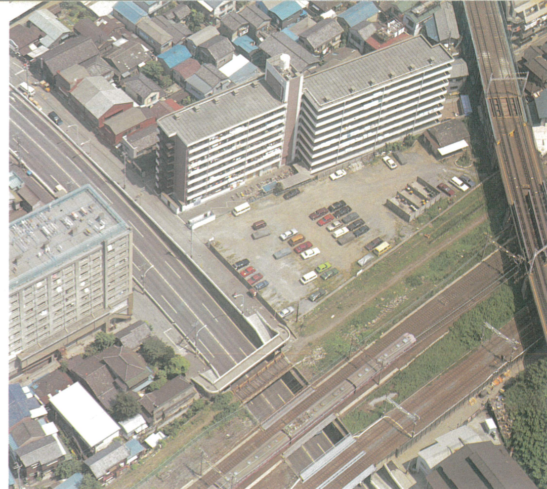
The Joban Line of the Japanese National Railways, which cuts through the southern part of Adachi Ward, is a vital transportation artery. 区の南部を走る国鉄常盤線は区民の大切な足だ。
